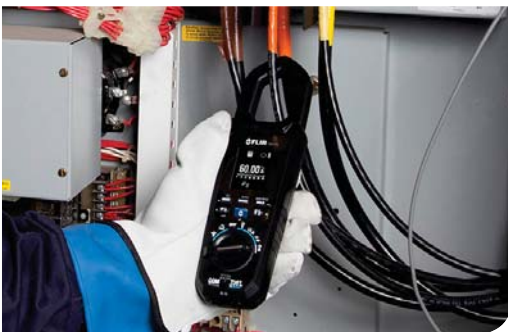
Verify amperage measurements
