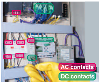
A mixture of AC and DC signals
