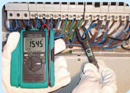
Measuring current in a Switchboard
