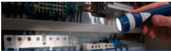
Erroneous circuit-breaker activation
